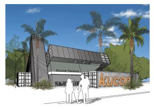
The concept plan for the Kucom Theatre provided a unique and extremely noticeable premises for a small amateur theatre company. Our concept used shipping containers as the primary structural form with economical sandwich panel infills providing the articulated roof form, niches for the required lighting rails and access walkways.
