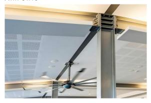
The introduction of low speed, high volume ceiling fans allowed an increase in the AC set temperatures, without any loss of comfort. Less cooling capacity was required, resulting in reduced plant and construction costs.
